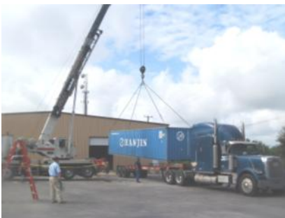
Loading container onto transport trailer.
