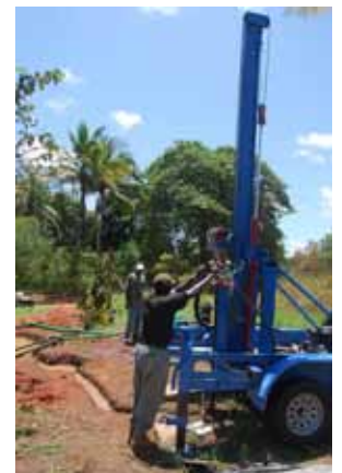
The drilling team uses new rig.
