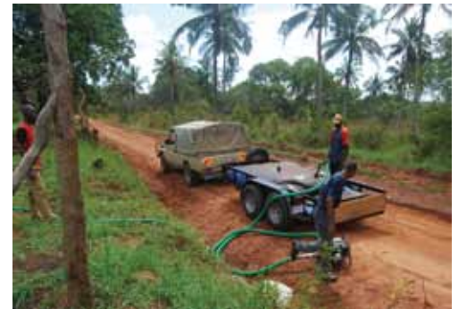
Crew pumps water for the mud pit.
