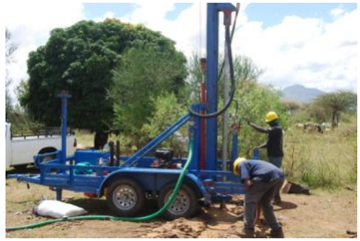
Geoffrey and crew trying to drill through rock.
