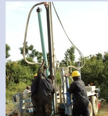
Ken helping drill for water
